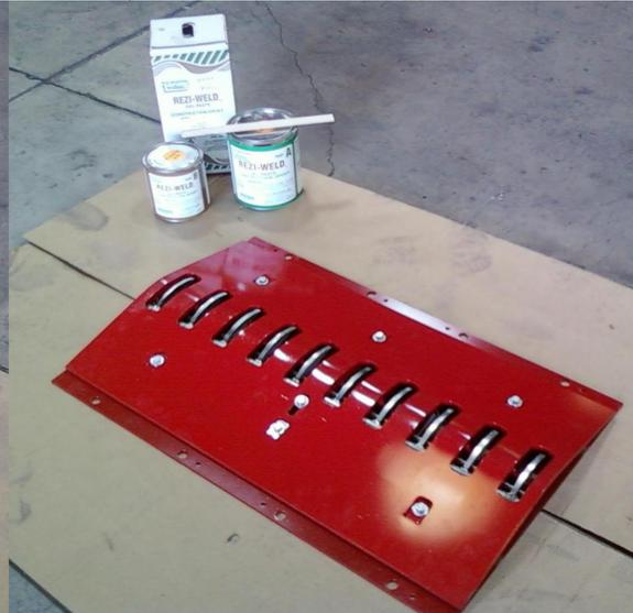
16. After all the toothed segments are installed, the end bevel sections (if used) can then be installed using the same procedure as the segments.
